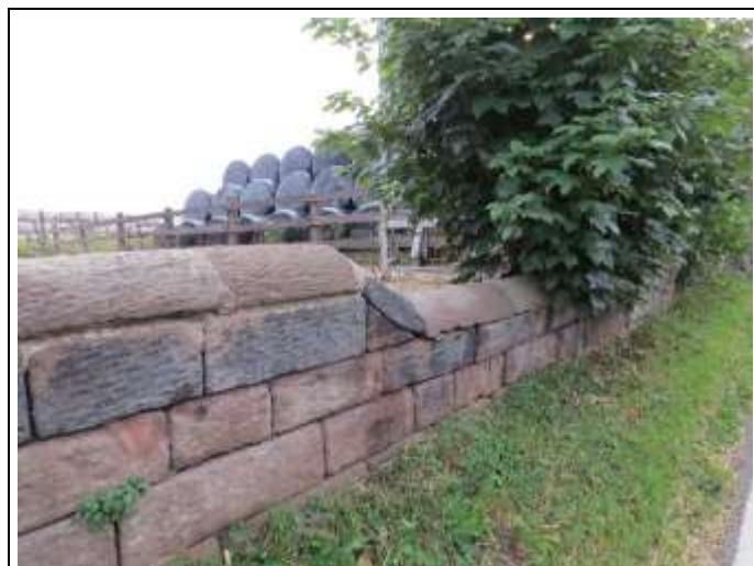
Boundary Wall of Farmyard
