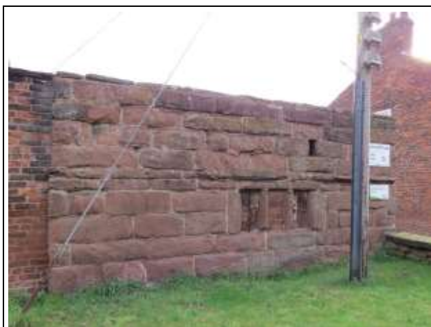
Squared Coursed Sandstone 17 th Century with Brown Brick to Either Side
