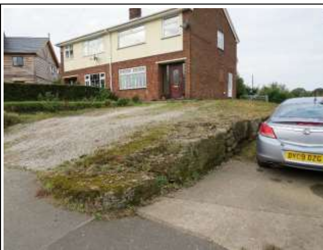
Stone Wall with Bedrock and Open Drive
