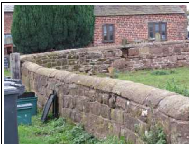
Boundary Wall at Hall Farm
