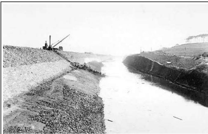
Construction of Ship Canal (Cheshire Image Bank)
