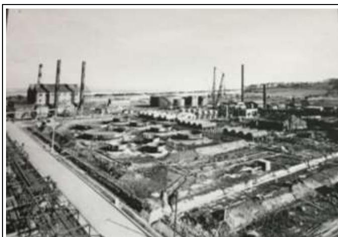
Construction of Stanlow Refinery 1940
