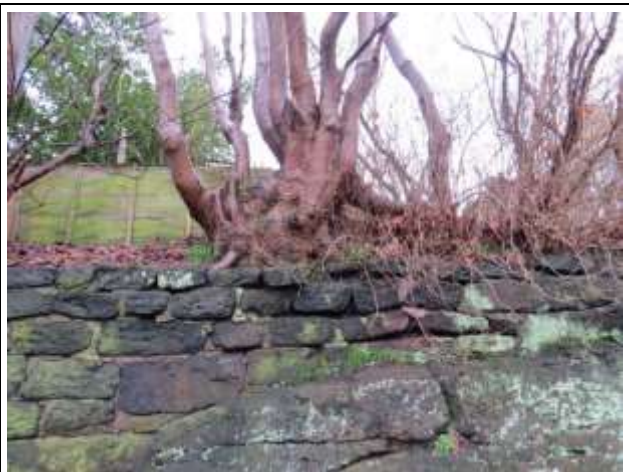
Stone Wall Incorporating Bedrock
