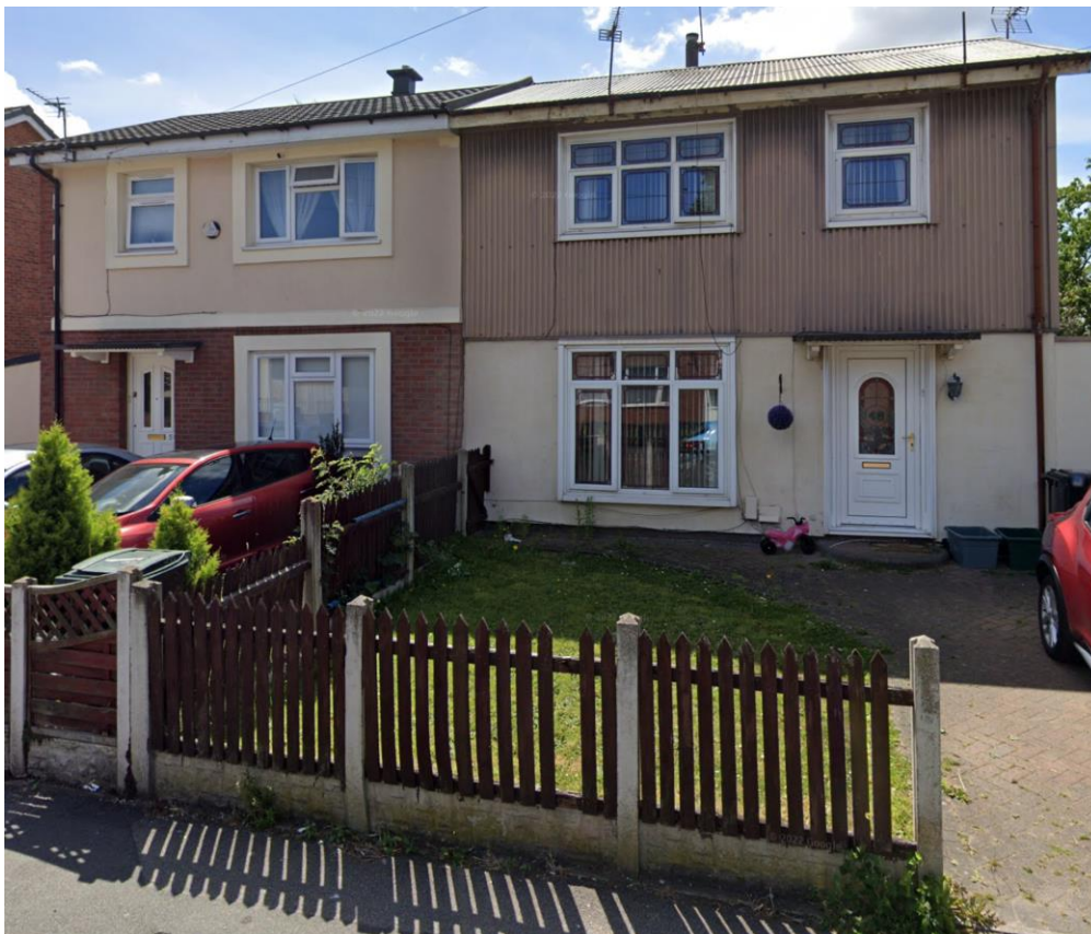
Typical unimproved BISF house (right) Council improved BISF house (left)
