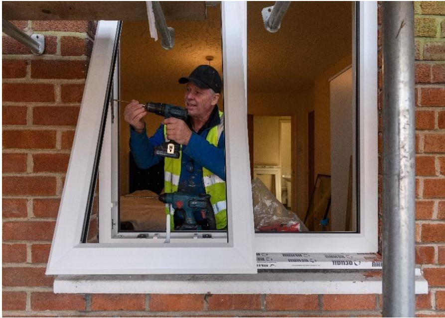
Window replacement programme
