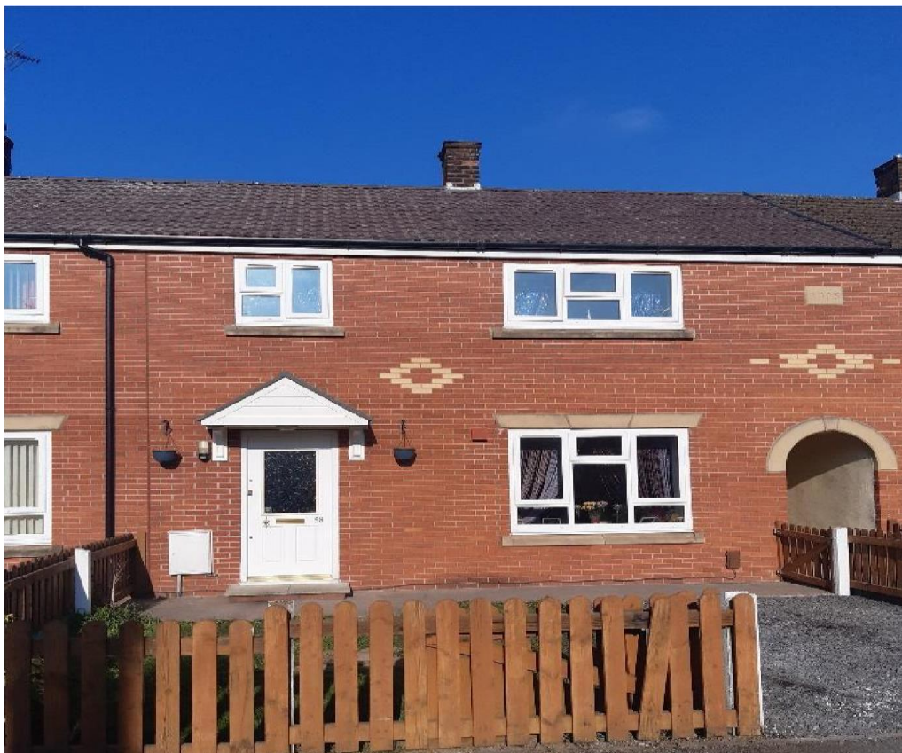
Typical roof refurbishment
