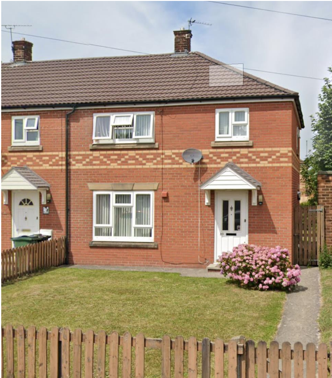
Typical Wates improved dwelling
