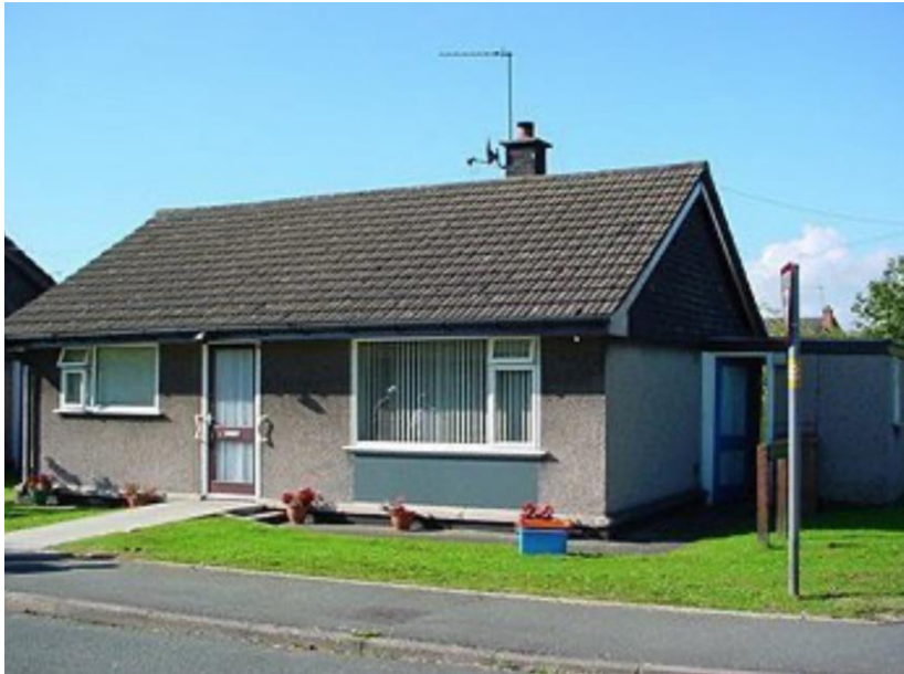
Typical Kencast Precast Concrete House
